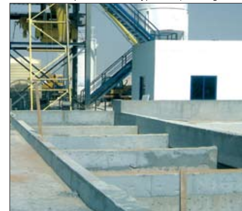
Silo en fila empotrado row type silo (below ground)
